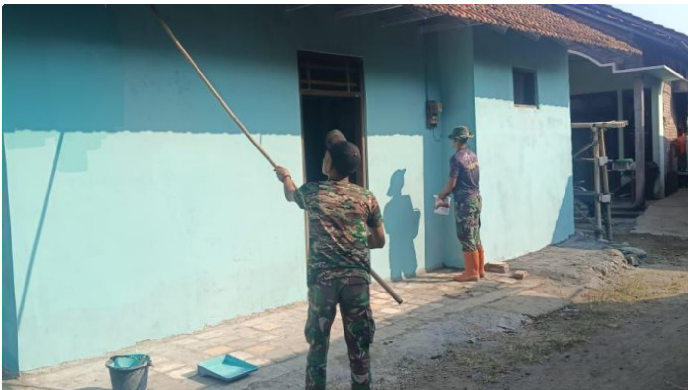
(Foto istimewa) Pengecatan RTLH TMMD 116 Kodim 0722/Kudus
